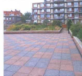
The day's third project was an intensive green roof sanctuary, where the Dreen tile was used to create pathways and communal areas surrounding a heavily planted area.
