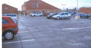
Car park in Newcastle, laid with Zoontjens' Pardak tile.
